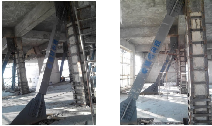
Figure 4.5.8 Strengthening site of the Military Museum Exhibition Building
